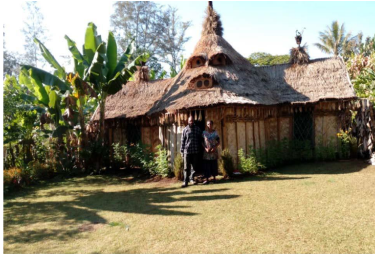
Figure 1: Newly built hut for arts and crafts
