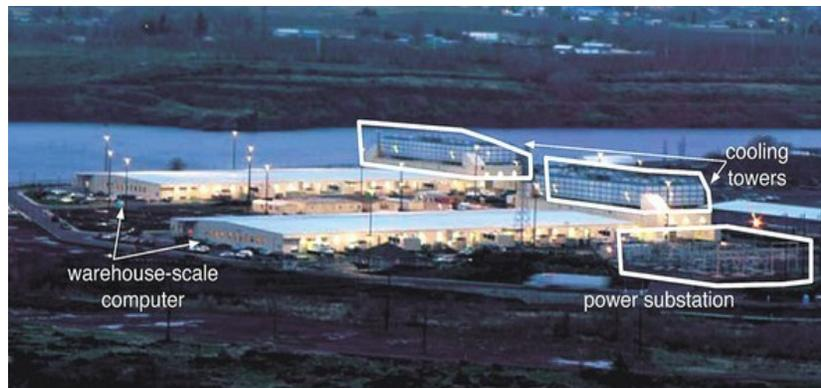
**Figure 15 Data center and warehouse scale computer**
